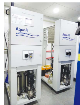
洗腎中心淨水系統 Water purification system of Renal Dialysis Centre
