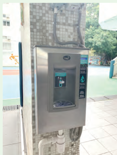
安裝斟水機取代舊式飲水機 Installing water bottle refill stations to replace with the old water dispensers
