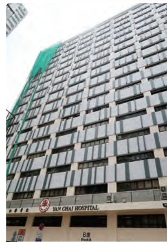
醫院外牆翻修工程 External wall refurbishment of YCH
