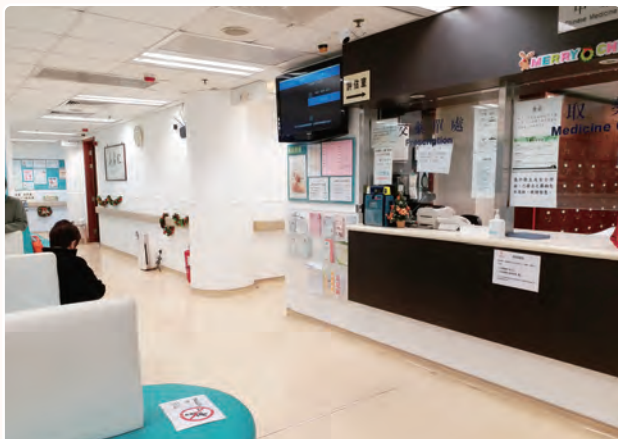
仁濟醫院—香港浸會大學中醫診所暨教研中心（葵青區）進行油漆翻新工程後，令診所環境更光猛舒適。 Renovation work has been completed recently at Yan Chai Hospital - Hong Kong Baptist University Chinese Medicine Clinic cum Training and Research Centre (Kwai Tsing District) for better environment to patients.
