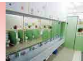
翻新後的兒童洗手間 Children's washrooms after refurbishment
